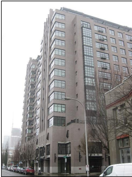
Photo A-3: Northeast elevation
