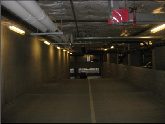
Photo A-11: Parking ramp
