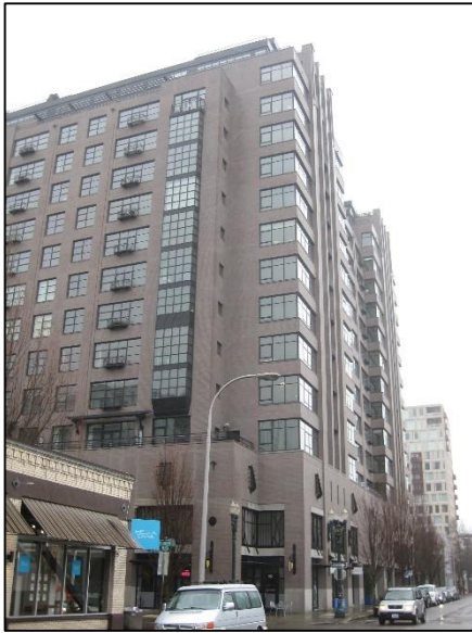
Photo A-1: Southwest elevation
