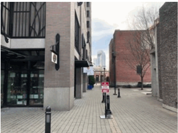
West side of building
