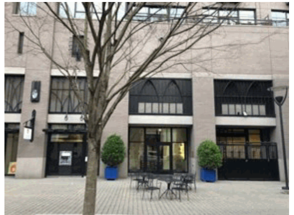
West side of building
